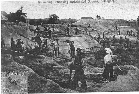
Tin mining: removing surface soil (Cheras, Selangor).
